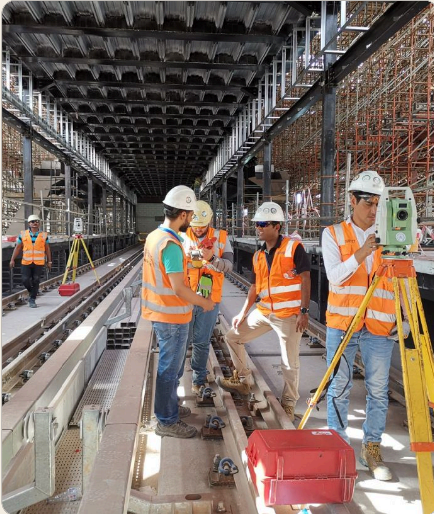
RIYADH METRO • TRACK SURVEY
